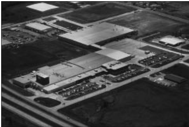
HEPI's Warrensburg plant covers 320,000 square feet and is situated on 33 acres
