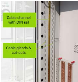
DIN Rail for breaker mounting.
