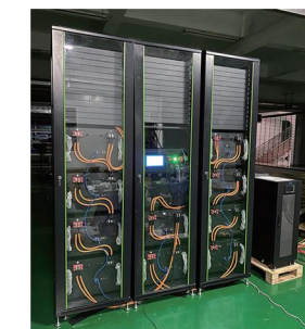
Network Computer Room
